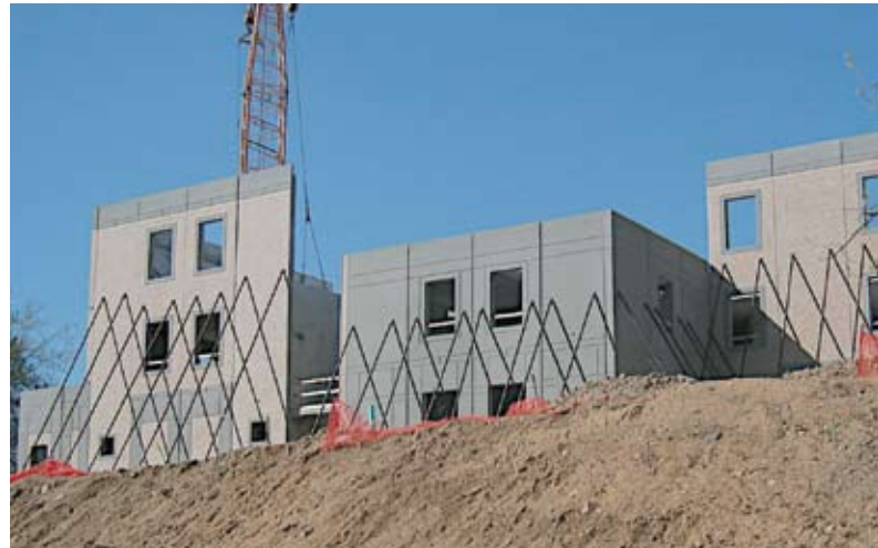
After being erected, the precast concrete panels are braced during construction of the Fairview Clifton school. Photo courtesy of Glaserworks.
